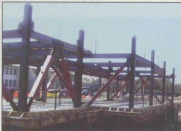
UNBONDED BRACE frames installed in a new building on the campus of the University of California at Davis are capable of withstanding several earthquakes.
